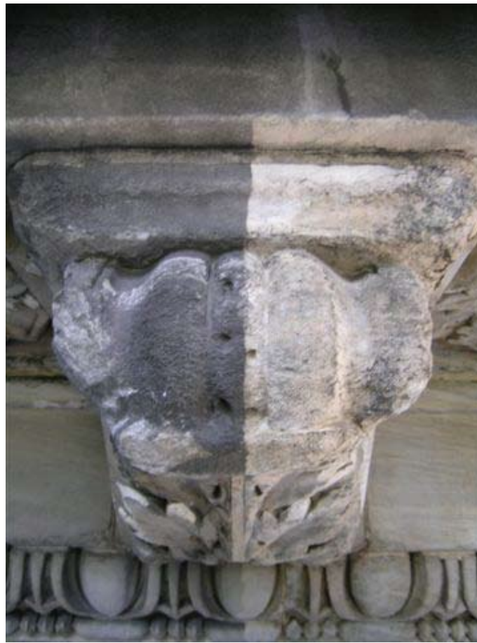
A balustrade before and after cleaning.
