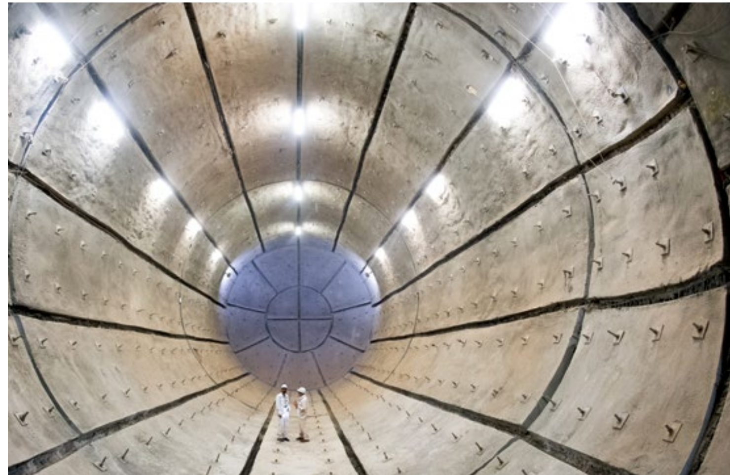
At Your Disposal Two men stand in the Konrad shaft nuclear repository being built in an abandoned iron ore mine in the city of Salzgitter in Germany. The deep mine will store low- and medium-level radioactive waste. As Richard Ovenden reminds us, “As a society we really need to be sure we will know long into the future ... exactly where we have stored nuclear waste, what material it consists of, when it was placed there, what kind of container it was stored in, and so forth.... Sound familiar? It’s called good archival practice.” PHOTO: JULIAN STRATENSCHULTE/PICTURE ALLIANCE VIA GETTY IMAGES
