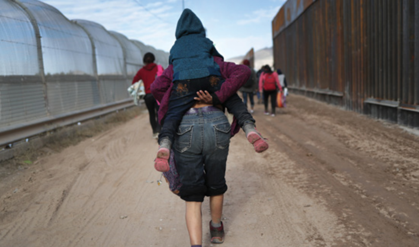
Fences After crossing the Rio Grande from Mexico into the U.S. at El Paso, Texas, Central American asylum seekers walk between a newly built “bollard-style” border fence, on the right, and the older “legacy” fence. They would later turn themselves in to agents from U.S. Customs and Border Patrol (CPB). PHOTO: JOHN MOORE/GETTY IMAGES
