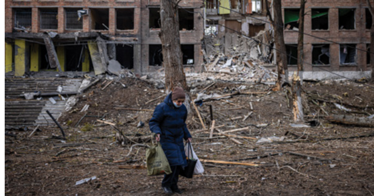
A woman walks in front of a destroyed building after a Russian missile attack in the town of Vasylykiv, near Kyiv, on February 27, 2022.
